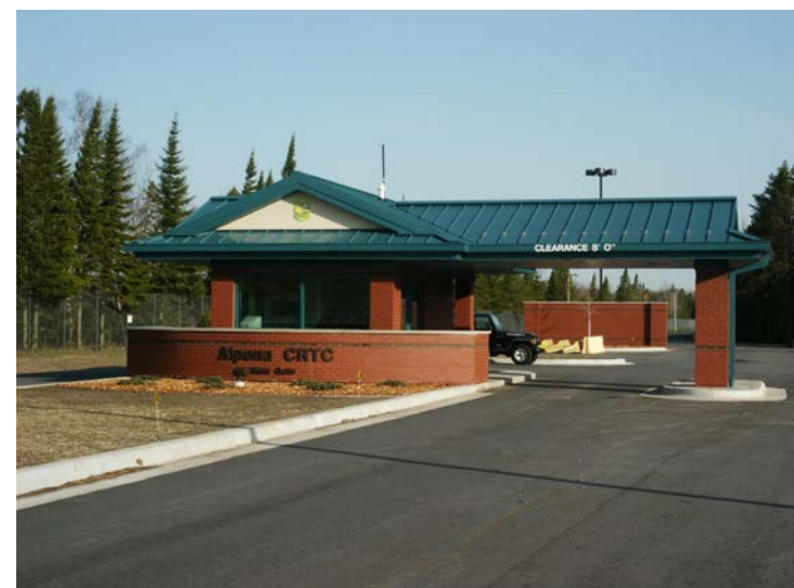
Front entry of Alpena CRTC, which is collocated with Alpena County Regional Airport. (Source: Alpena CRTC Public Affairs)
