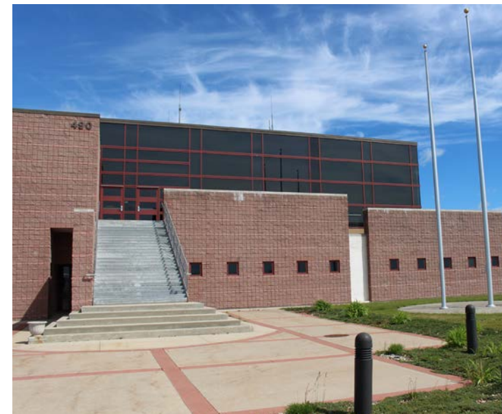
Base operations building.
